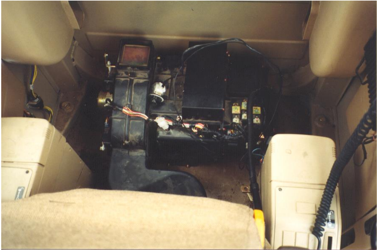
Evaporator/Heater assembly in place with thermostat inserted
